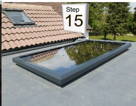
Beware, once frame is clipped down it can not be removed. If this needs to be done see next step, more clips will be required.
