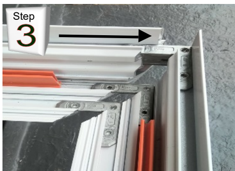
On a flat base (the glass panel is ideal for this) join the frames.
