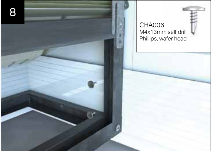
Fix the vertical frame into the fascia board using 2x CHA006 (M4 x 13mm) self drill Phillips, wafer head screws (supplied).
