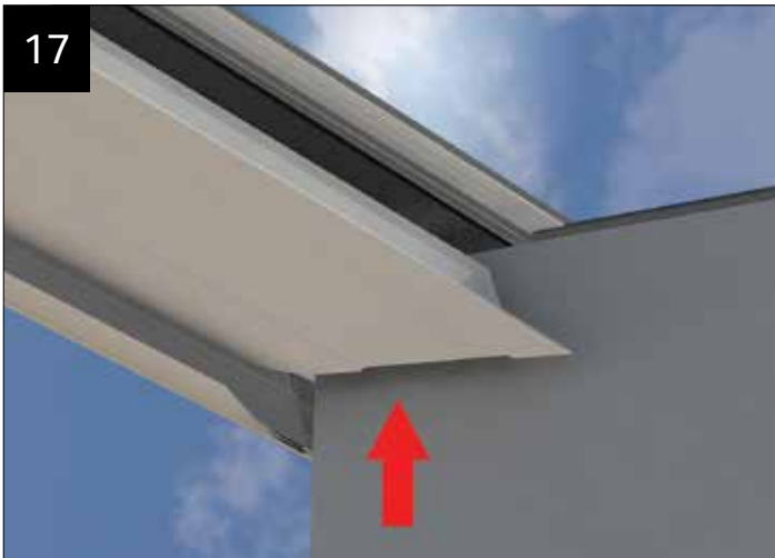
Classic Plus Valley cladding being fitted against pelmet. After plasterboard and skim.
