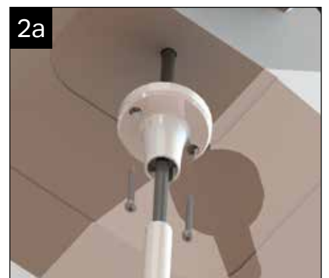
2a Offer up the internal radius end cap, retain this using the tie bar ridge fixing cover and two self tapping screws provided. Cut the PVCu conduit to suit.
