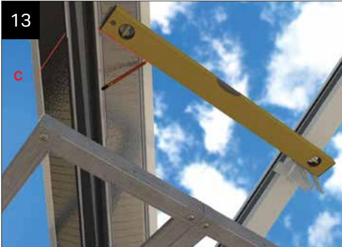
Using the bracket positions, level through and mark off the valley marked 'C'.
